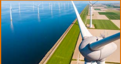
An aerial view of the Westersemeerdijk wind farm in the IJsselmeer, the largest wind farm in the Netherlands.
