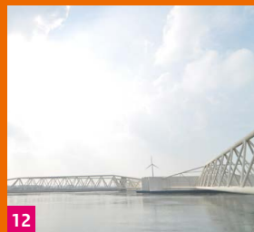
The Maeslantkering is the largest moving flood defence in the world. The flood defence system closes to protect the land when the sea rises due to a storm. (p. 7)
