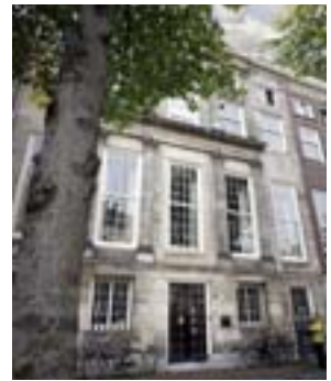
page 17 Herengracht 410-412 Amsterdam Built in 1644 Architect: Philips Vingboons
